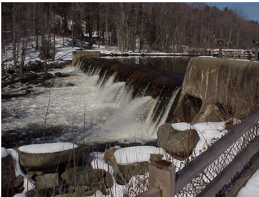
Figure 2 – Photograph of Wiswall Dam
